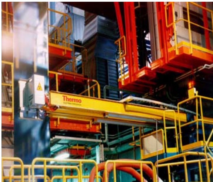
Zinc Coating gauge in operation
