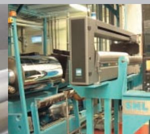
Scanner Installation on Line 4
