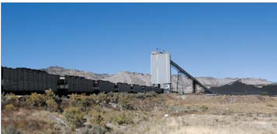
Figure 10. The north rail loadout capitalises on the sorting ability of the mine coupled with another coal analyser on the loadout conveyor.
