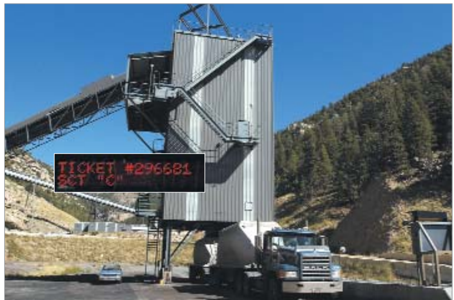
Figure 6. Up to 350 trucks/day haul 43 t each to one of two rail loadouts, with their actual stockpile destination at each loadout determined by the real-time analyser results. The scoreboard (inset) provides this information immediately upon completion of the truck loading.
